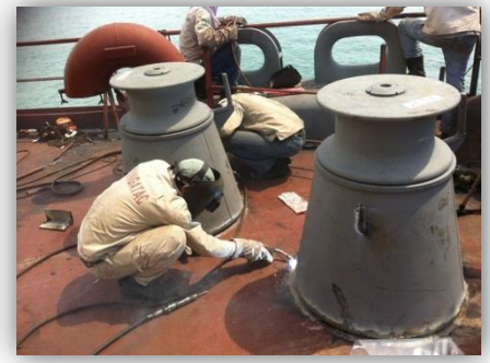
Installation of Mooring Arrangement
