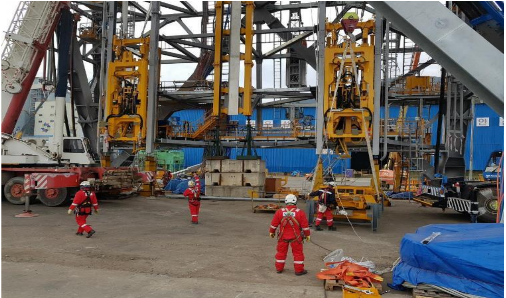
Reference Photo – Derrick Assembly
