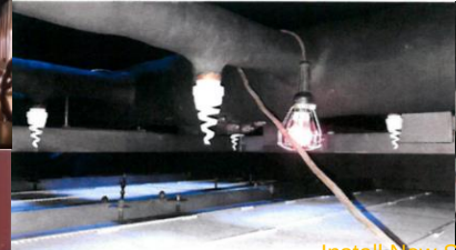
Install New Scrubber Sprayer
