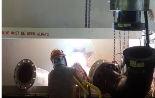
Shipside Distance Piece Repair -Outside
