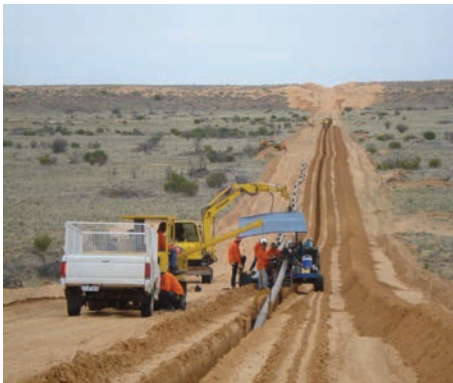
Spinner and crew laying in the pipe
